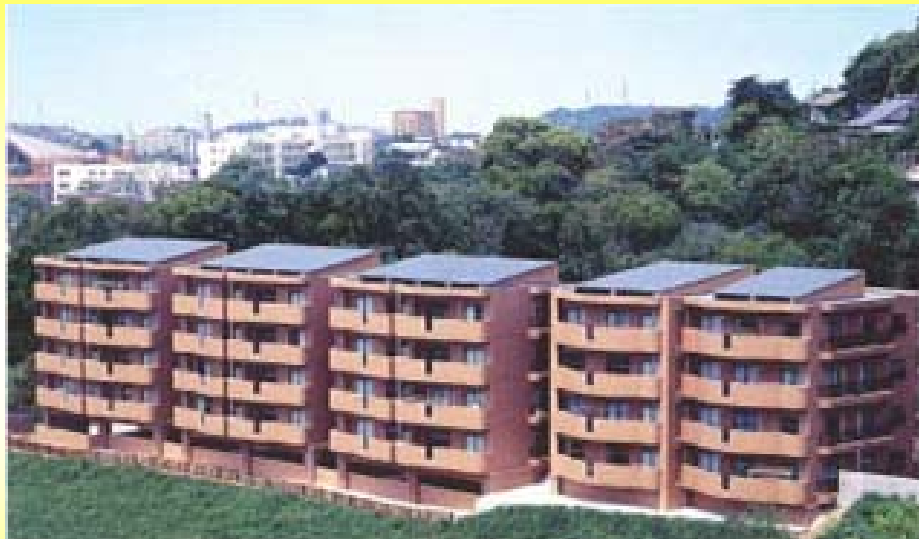
PV Power Generation 51kW (300W × 17units)
